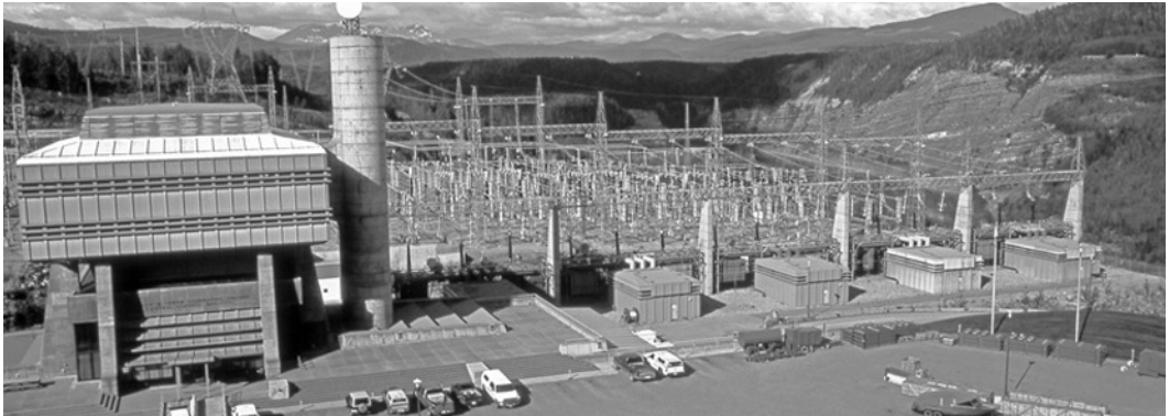
Figure 5. Environmental inventories and assessments for construction of the W. A. C. Bennett dam west of Hudson's Hope, BC in the mid-1970s provided new information on bird-use of the Peace River. Photo by R. Wayne Campbell, 15 June 2003.
