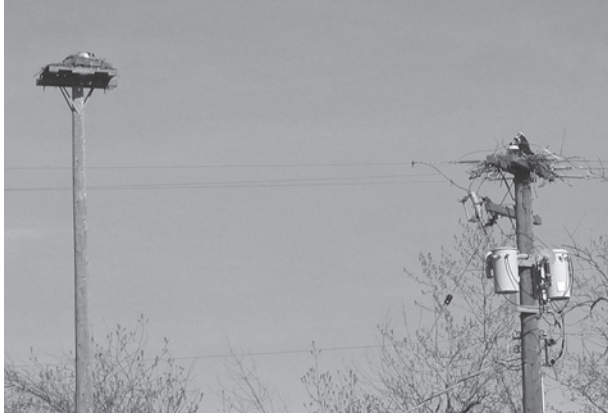
Figure 68. Poles with no electrical current are often installed so Osprey have a safe site on which to build their large stick nests. Canada Geese are also attracted to these elevated sites which force the Osprey to build a new nest, often on energized poles. Near Creston, BC. 23 April 2005. (Cyril Colonel).
