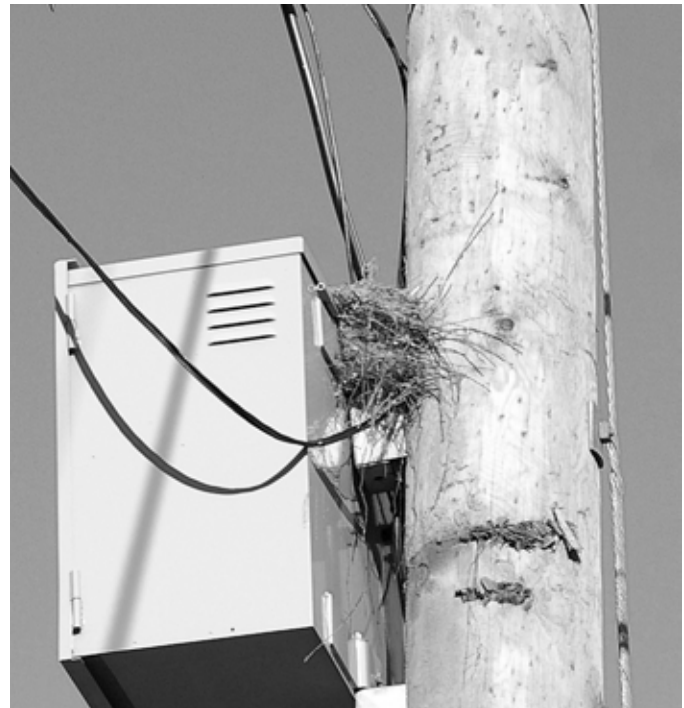
Figure 84. Most Western Kingbird nests reported in British Columbia are built on wires and metal supports behind transformers attached to telephone poles. Photo by Vicky Atkins, Vernon, BC, 5 July 2012.
