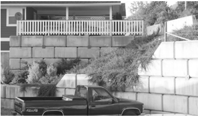
Figure 186. Northern Rough-winged Swallows have recently taken advantage of nest sites provided by concrete retaining walls in urban and residential areas. Photo by Gary Breault, Creston, BC, 27 July 2012.
