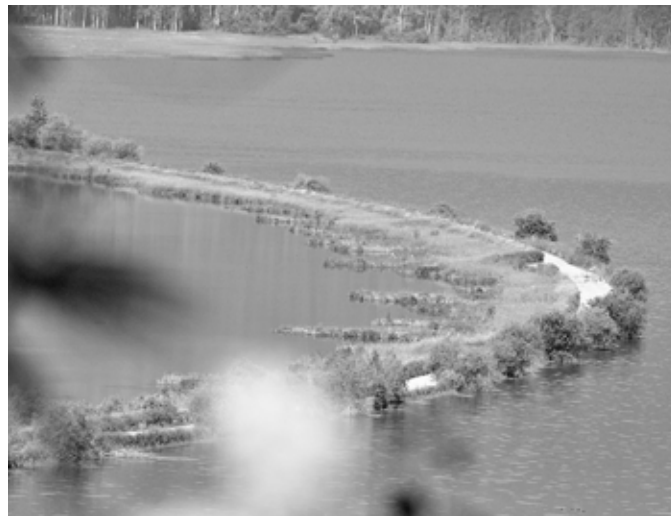
Figure 143. View of a portion of Duck Lake from highway 3A. The rising water posed a threat to the main road access along the dyke at the lake. As a safety precaution, the dyke was inspected by an engineer before re-opening for public use. Photo by Linda M. Van Damme, 8 July 2012.
