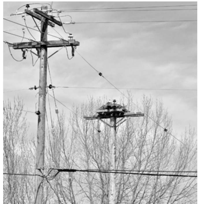
Figure 162. A new de-energized pole installed in 2011 by FortisBC in West Creston was adopted by a pair of Osprey in the 2012 season. The supporting structure was complete with its own insulator. One young was observed at this new nest site but did not survive to fledging stage. Photo by Linda M. Van Damme, Creston, BC, 20 April 2012.
