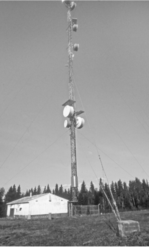
Figure 17. Telecommunication and broadcasting towers, usually tall structures built on high points of land, may require access roads for maintenance, spraying to control vegetation, and stream crossings. Photo by R. Wayne Campbell.
